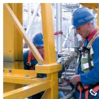
Service for air cargo terminals
