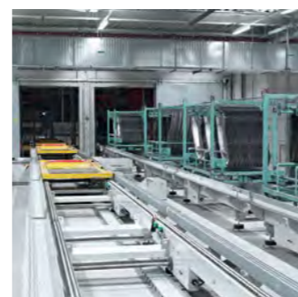
Material handling system (BMW Group, Workshop Dingolfing)
